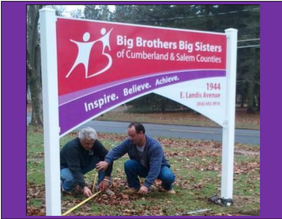
FALASCA MECHANICAL WORKERS INSTALL LIGHTING ON THE NEW AGENCY SIGN
